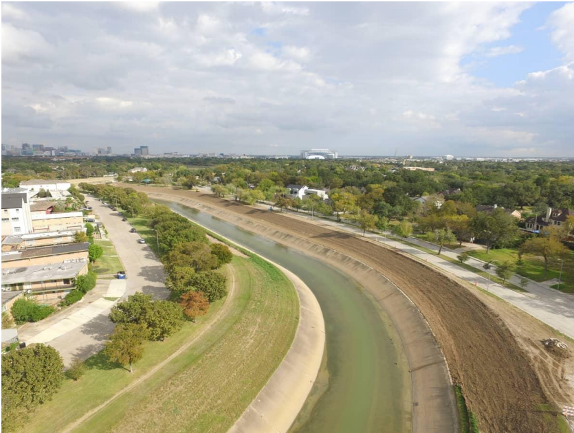
Brays Bayou Federal Flood Control Project Channel Modifications Discrete Segment 109 - $12,340,249
