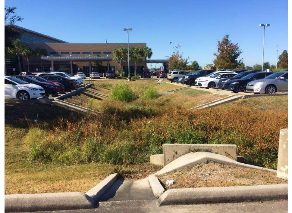
FLOOD MITIGATION PROJECT, ST. BERNARD PARISH
