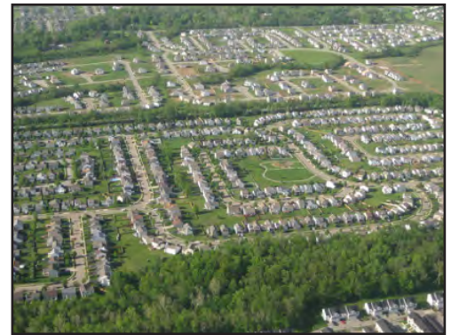
A low-density, American suburb. Single-family subdivisions across the Capital Region such as these generate significant vehicular traffic, especially at one-way entry and exit points and utilize municipal infrastructure inefficiently.
