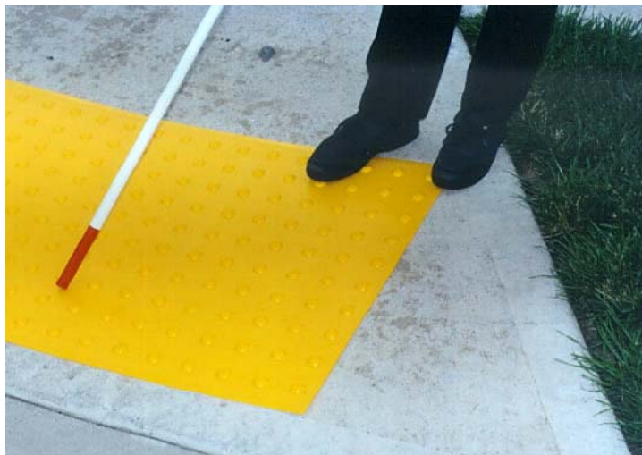
Tactile and contrasting color detectable warning strips provide pedestrians with vision impairments and important queue that they are leaving the sidewalk and entering a street.
