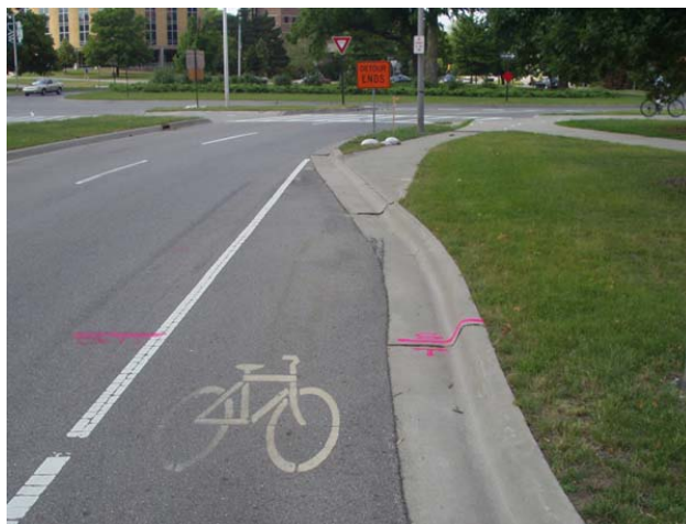
A ramp that eases the transition from a Bike Lane to a Shared-use Path is provided where the Bike Lane ends.
