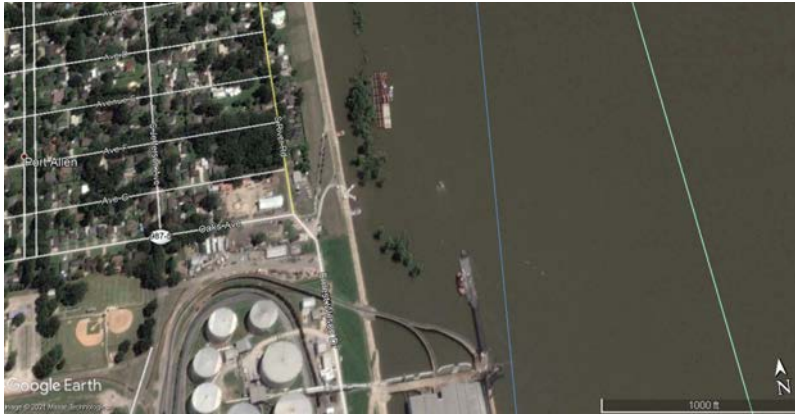
FIGURE 67 – PORT ALLEN OAKS AVENUE AT FLOOD LEVEL
