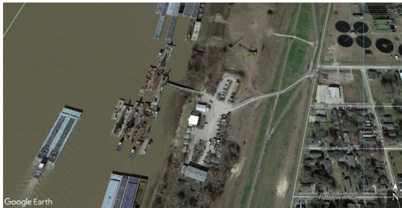
FIGURE 75 – LSU MCKINLEY STREET (E5)
